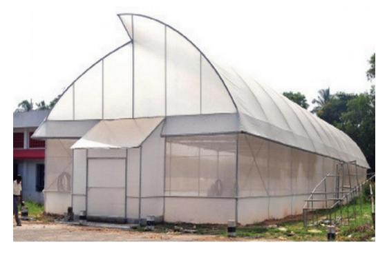
Polyhouse is a structure made of translucent material like polyethylene where the crops grow and develop under controlled climatic conditions. In developing countries like India polyhouse is a popular greenhouse technology due to its low cost of construction and easy maintenance. Polyhouse is cheaper as compared to greenhouse but the latter is more long lasting than polyhouse.
